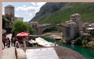
Stari most / Old Bridge
