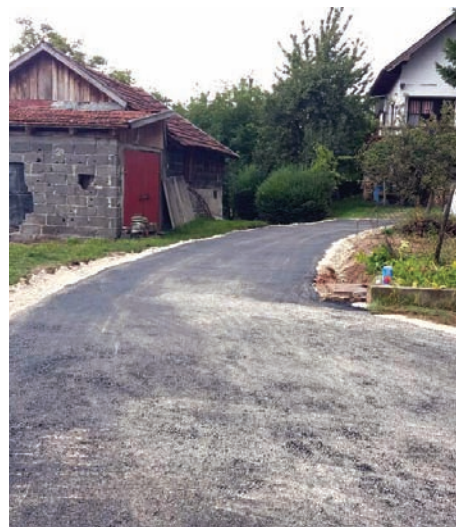
Hladivode pristupni put
